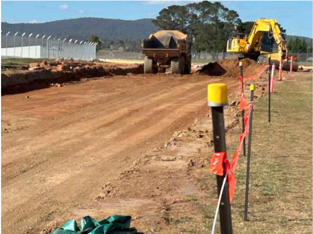
Photo 2: Earthworks in progress for the Northern Road (photo taken 21 Feb 2025)
